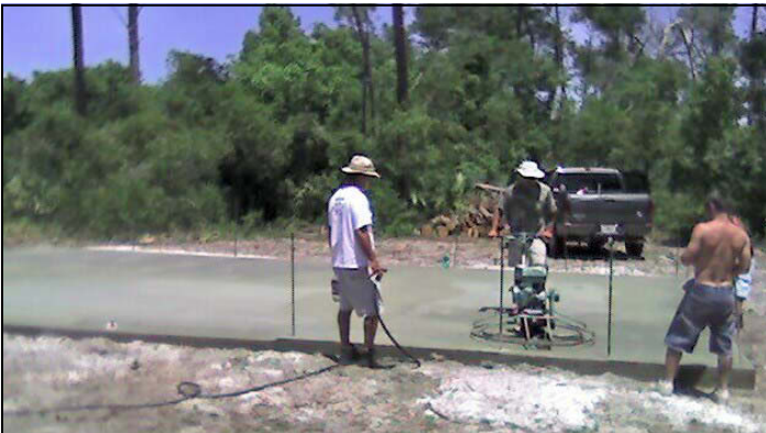
Final work being done on the slab.
