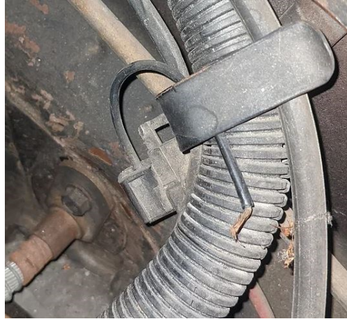
Wire Lead @ Driver Side Fire-Wall
